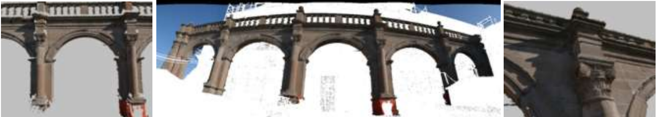
Fig. 2: geometric description of arcade with laser-scanner
